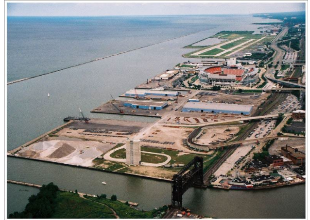
Coke, Ontario Stone Corp., Sand Products, Shelly Company, and St. Mary's Cement.
