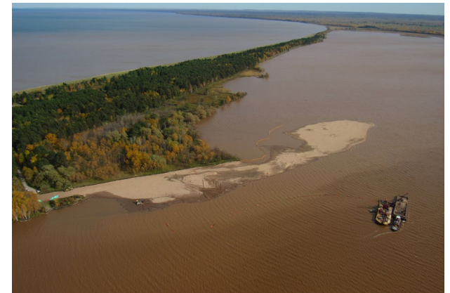
Shallow water placement for habitat restoration using dredged material Superior, WI
