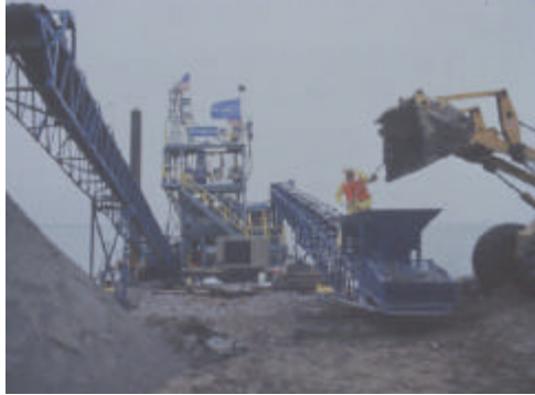
Fig.4 ARCS Physical separation technology demonstration at Saginaw, MI
