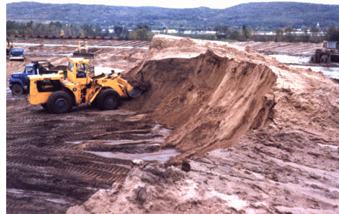
Figure 13. Washed sand at Erie Pier CDF in Duluth
